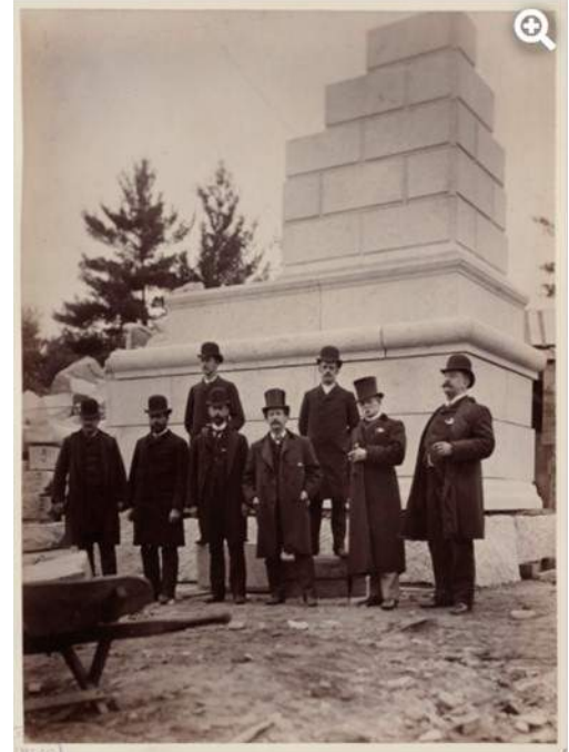
Dignitaries pose in front of mock-up cornerstone for the McKim Building assembled at the Milford Quarry.
