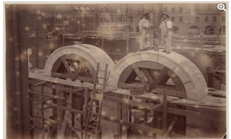
Arches for entrance to courtyard from Boylston Street entrance, construction of the McKim Building
