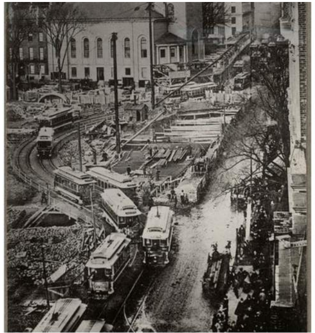
Subway construction at Park Street Station, Boston, Mass, circa 1895-97
